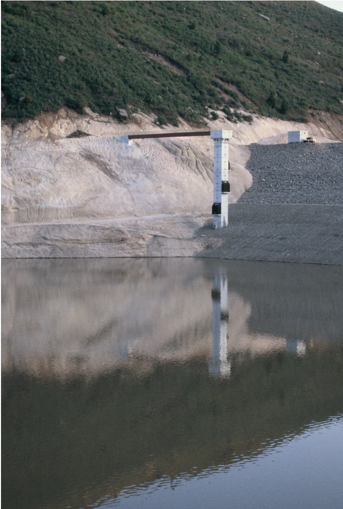
Figure 15. Selective Outlet Works showing the 2nd and 3rd outlets. The 1st outlet faces the dam. Note the proximity of the 3rd SLOW to the benthos.
