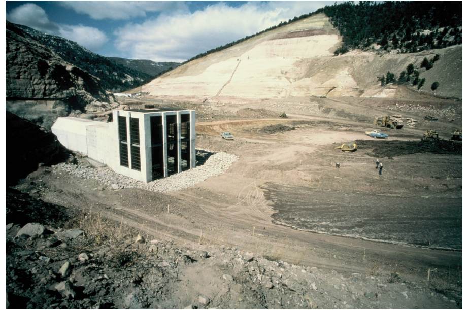
Figure 16. Gates at bottom of reservoir. Dam has not been constructed.
